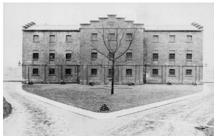
Allegheny Arsenal Laboratory Building (circa 1870) and the Stone Road
